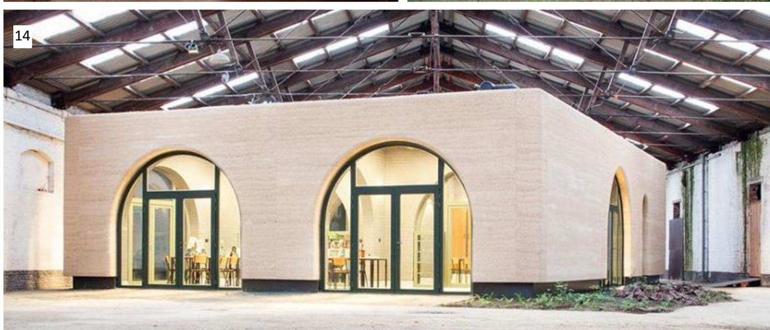
1. **L'ORANGERIE DE LYON CONFLUENCE**, LYON, 2021, ARCHITECTE : FABRICE FOUILLET & CLÉMENT VERGÉLY ARCHITECTES, (PISÉ PORTEUR PRÉFABRIQUÉ ET OSSATURE BOIS INTÉRIEURE (9 M))
