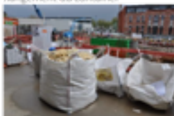
Installation zone de tri (photos : OCB-C & CSTC)
